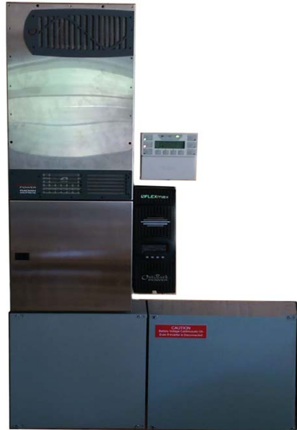
CPS Energy Storage System 4kw/10kwh
